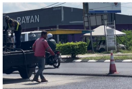
Figure 3. Cone protection was tested during road maintenance work
