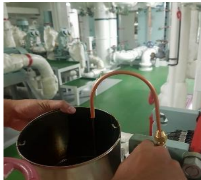
Figure 8: Smooth Drain of MDO Fuel Source: Authors
