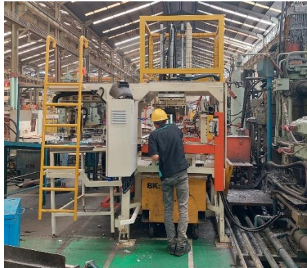
Figure 6 Automated trimming press insatalation process
