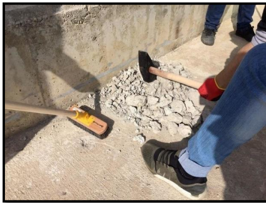
Figure 2. Construction waste that crushed to fine aggregates size
