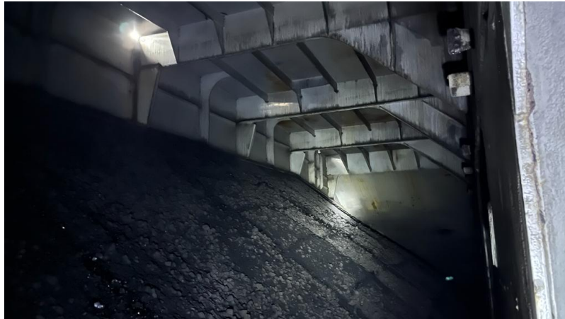
Figure 2. Broken Space in Hatch No 2 Source: Researcher Document (2023)
